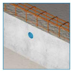
9) The CSD® fixation pieces that are affixed to the formwork can be re-used for subsequent projects.
